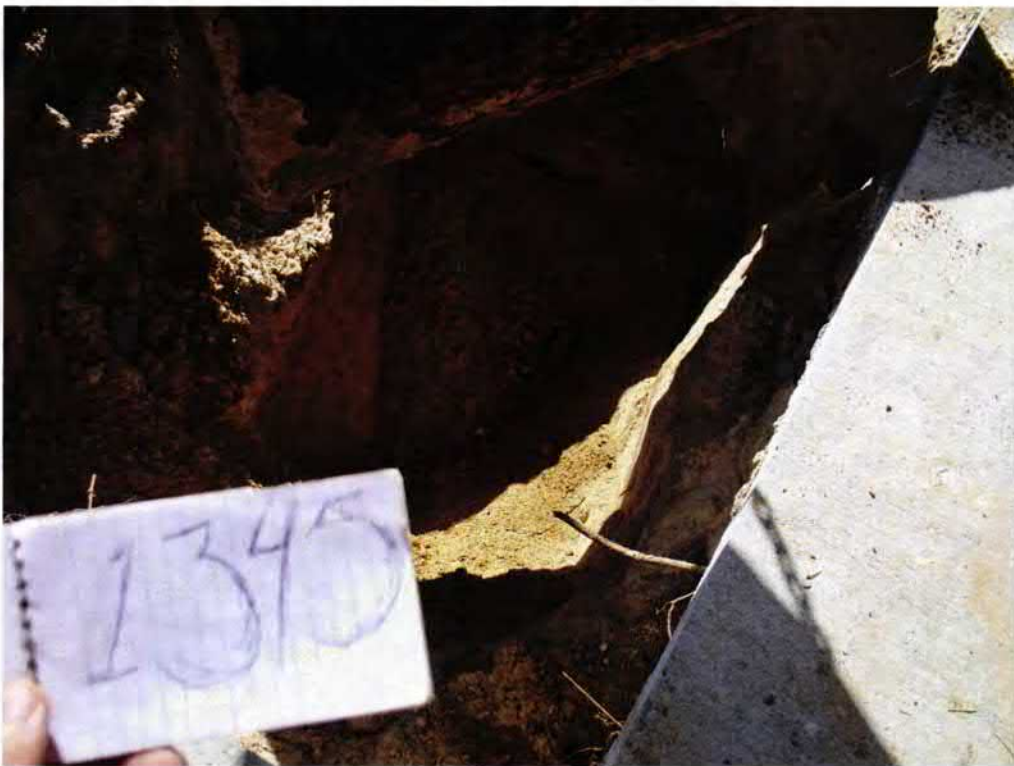
Picture 2: UST 1345 Cardinal excavation.
